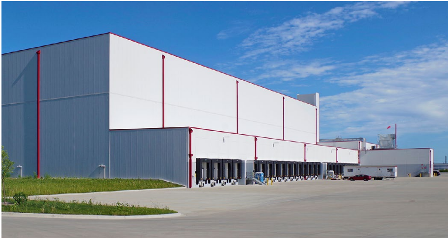
An example of a gateway distribution facility in Romeoville, Illinois.
