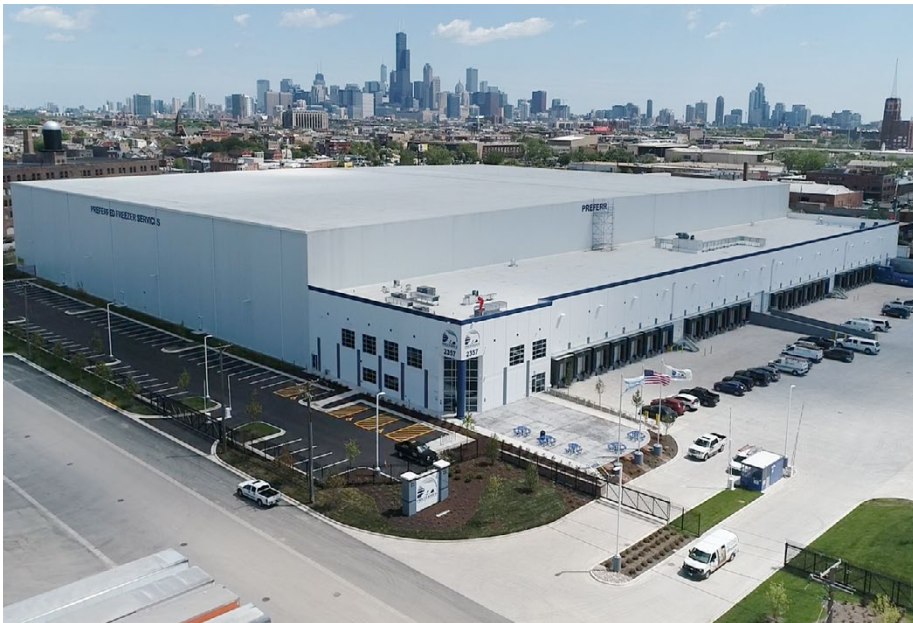
A regional cold storage distribution facility outside Chicago.
